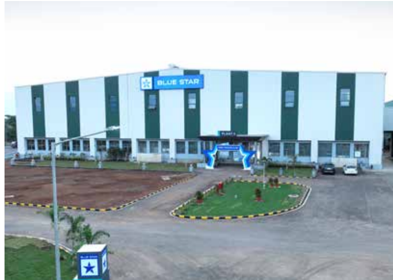
Wada – Deep Freezer Plant
